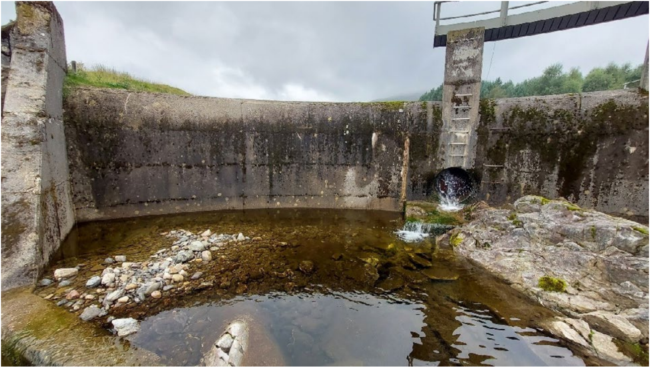
Figure 5.9. Concrete dam on RoR Case study three, illustrating a small orifice low in the structure. Photograph looking upstream.
