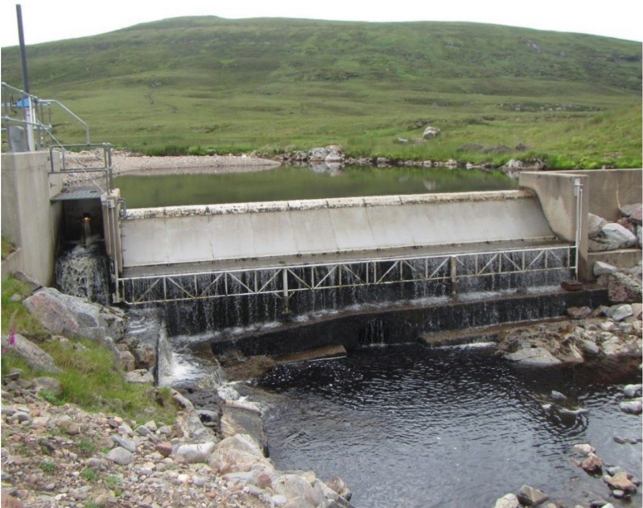
Figure 5.5. RoR Case study Two intake structure . Photograph looking upstream.
