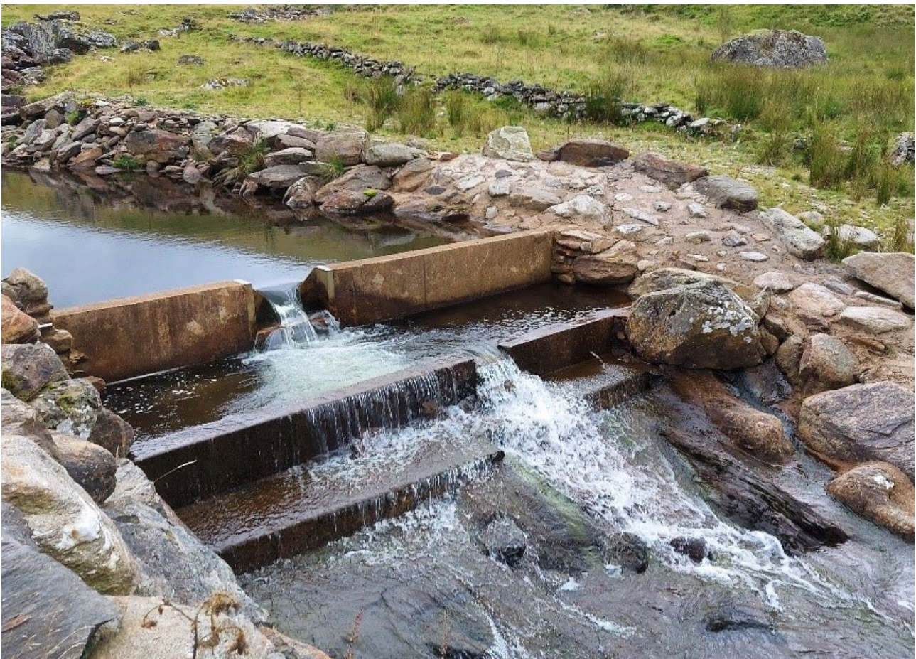
Figure 5.13. RoR Case study Four impoundment illustrating multiple small, notched structures. The upper v-notch is approximately 1 m-wide and the two steps are 0.5 and 0.25 m high. Photograph looking upstream.
