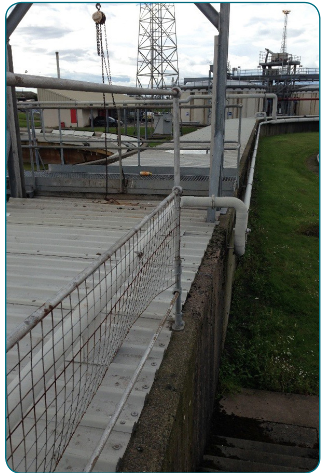
Figure 4: Covering on channel from inlet works to primary tanks
