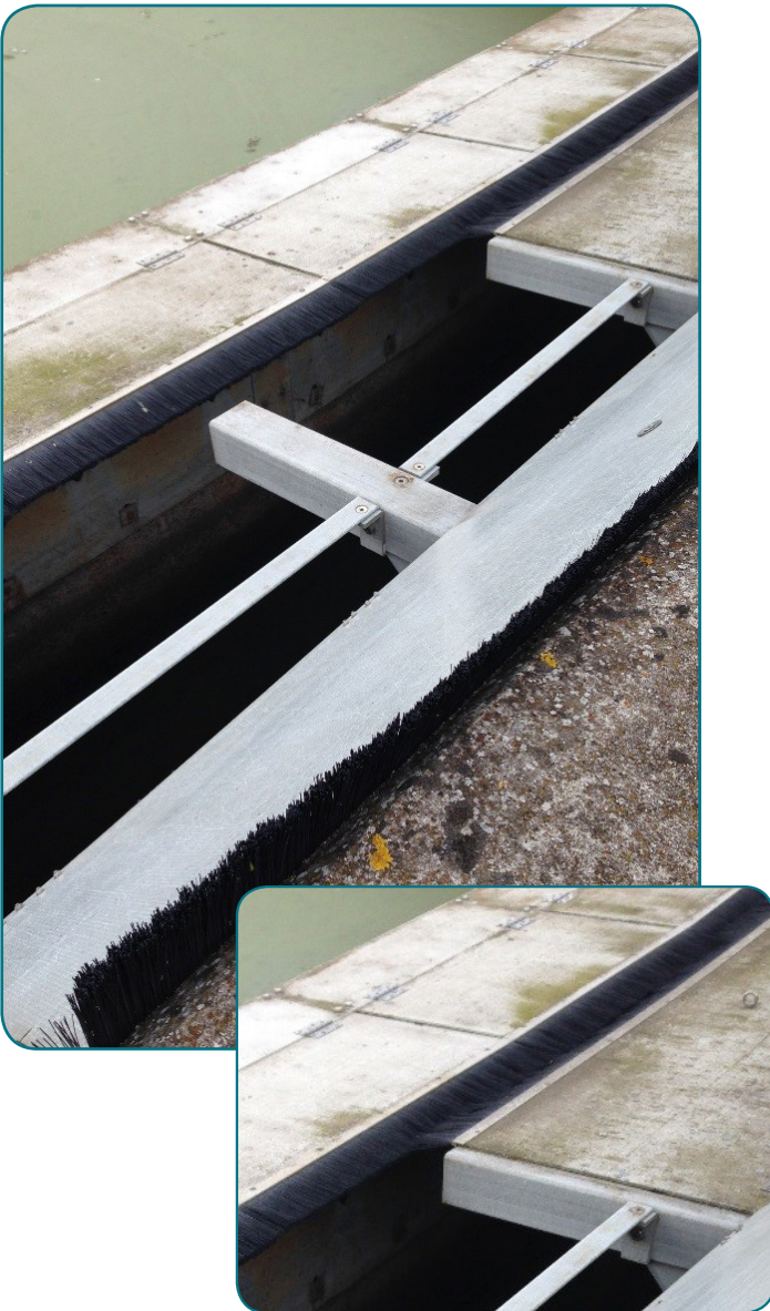
Figure 3: Brush covering on primary tank weirs
