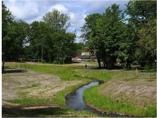
Figure 6 - De-culverted Tollcross Burn
