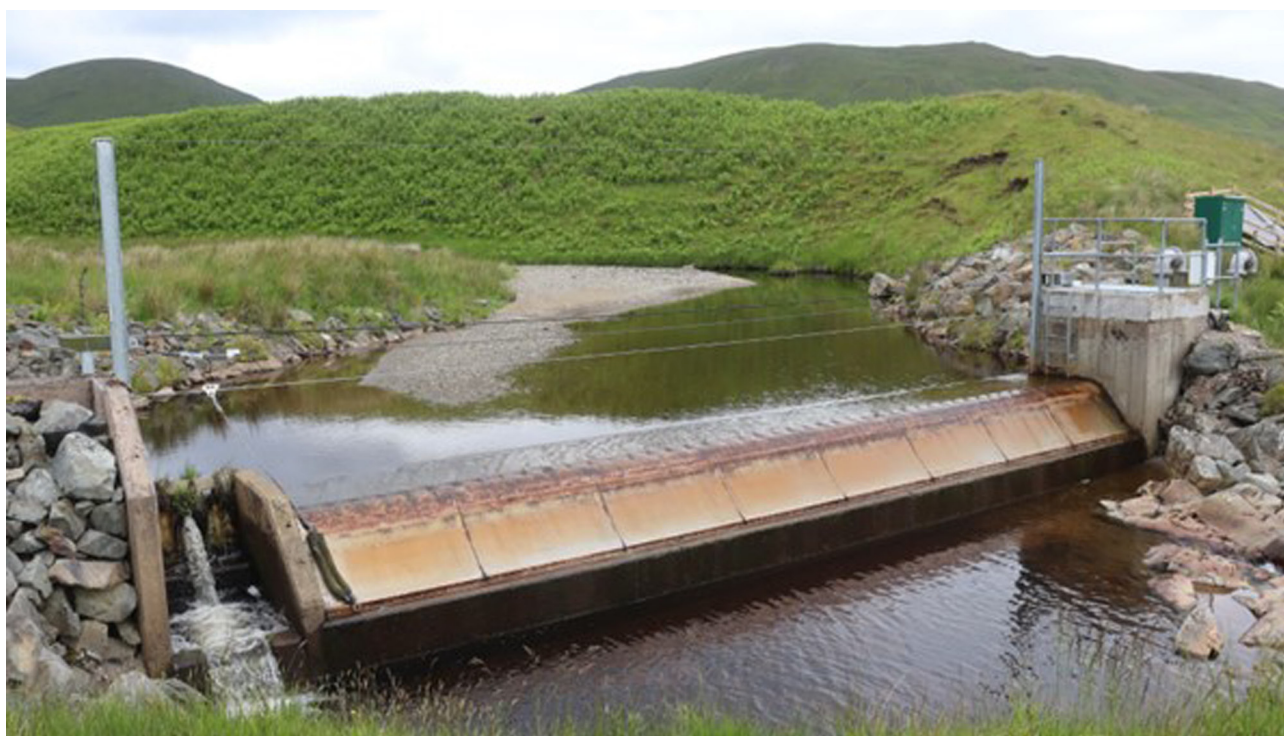
Figure 1 – Hydro impoundment (Photograph courtesy of Richard Williams).
