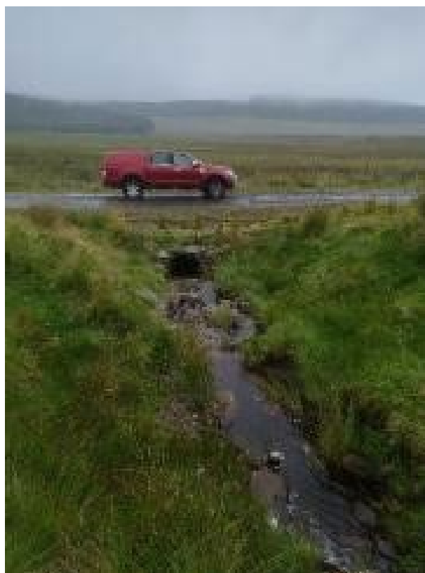
Figure 7. Culvert maintaining surface water flow.
