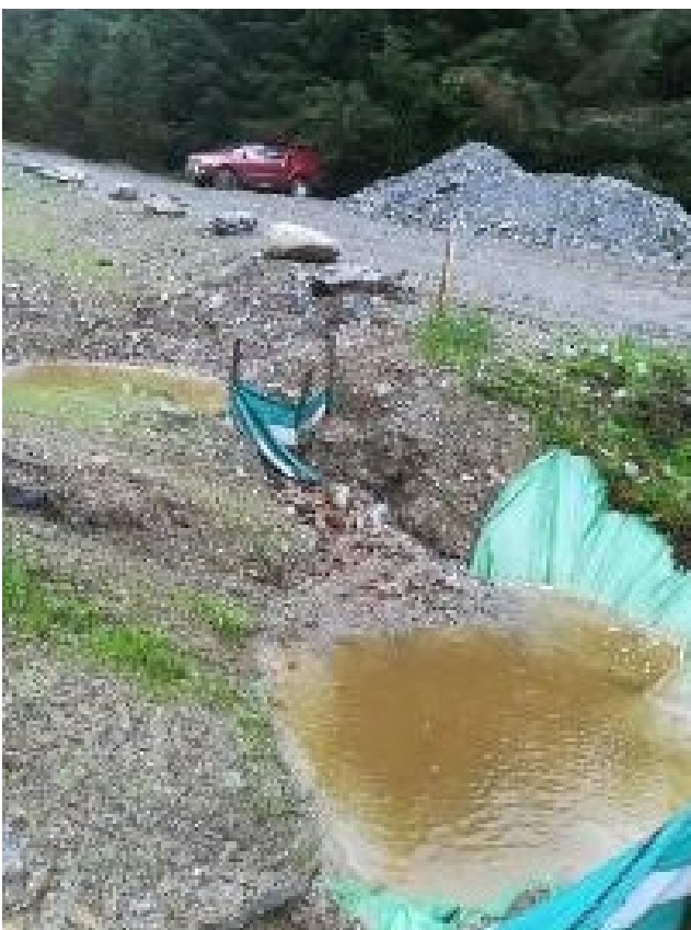
Figure 4: Left panel: Silt-trap. Right panel: Silt trap out of line with culvert.
