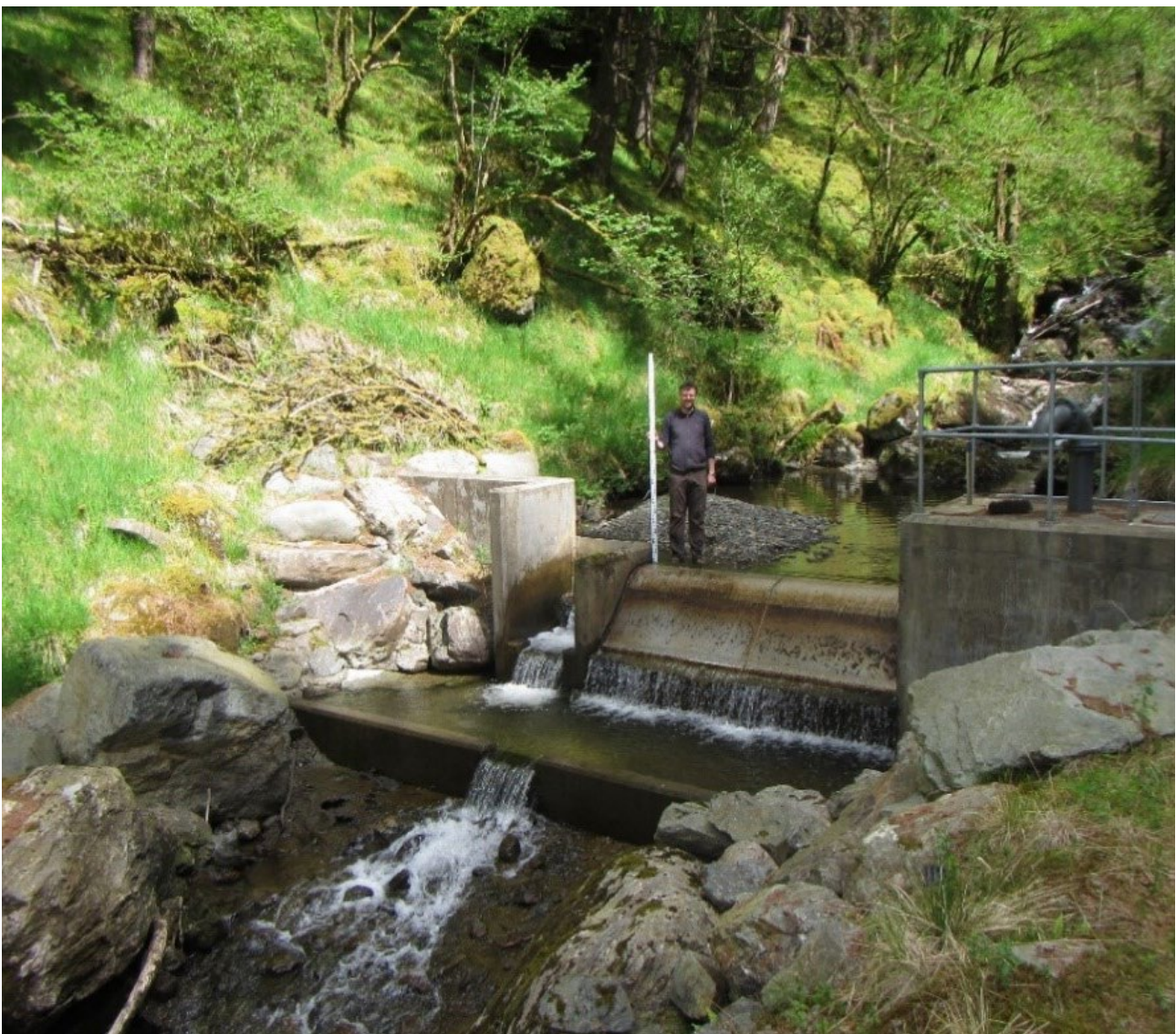
Figure 5.1. RoR case study One, hydropower scheme intake and weir. Note the sediment deposit in the headpond.
