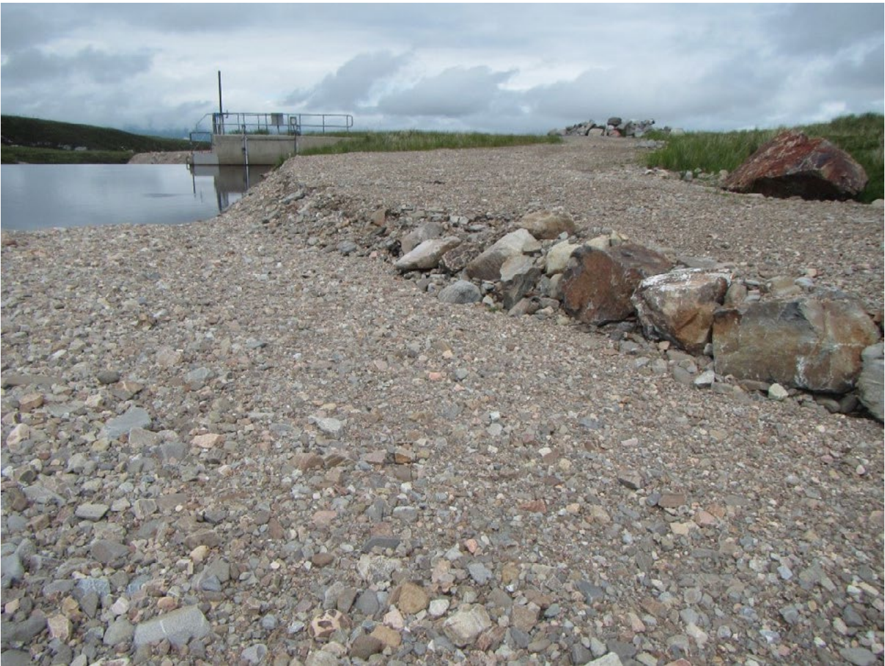
Figure 5.8. Pavement built on the right bank of the headpond of RoR Case study Two, using dredged material. Photograph looking downstream.
