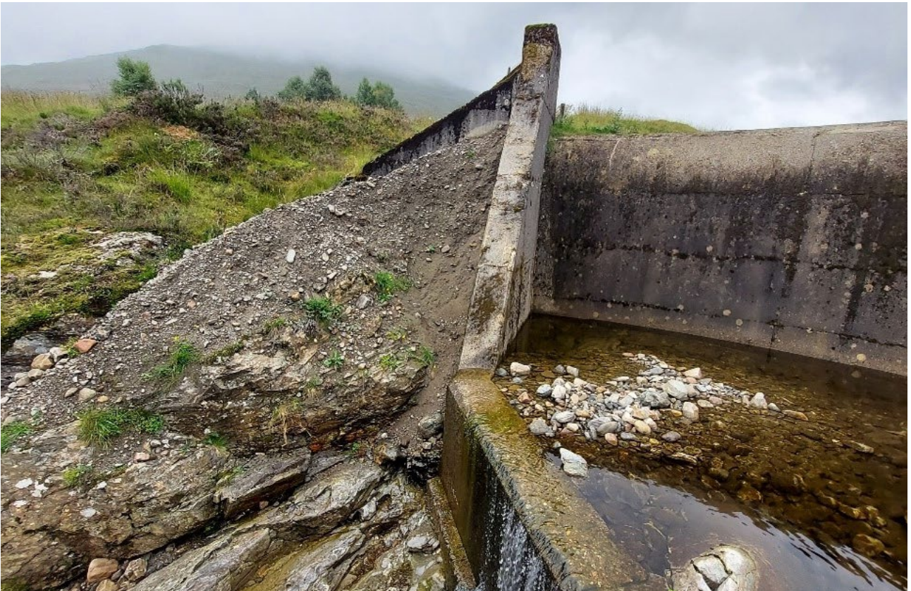
Figure 5.11. Mechanically reallocated sediments on the river right bank (left side of the picture), just downstream of the impoundment.
