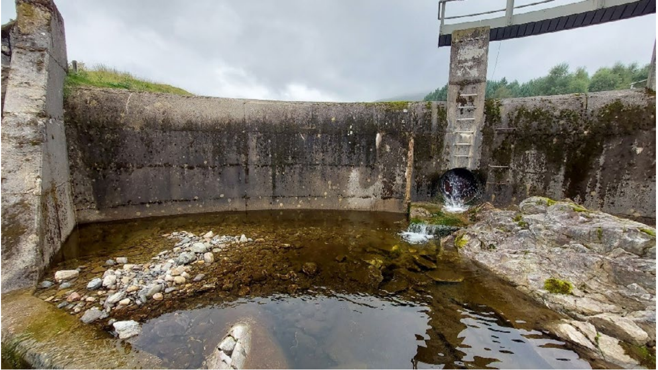
Figure 5.9. Concrete dam on RoR Case study three, illustrating a small orifice low in the structure. Photograph looking upstream.
