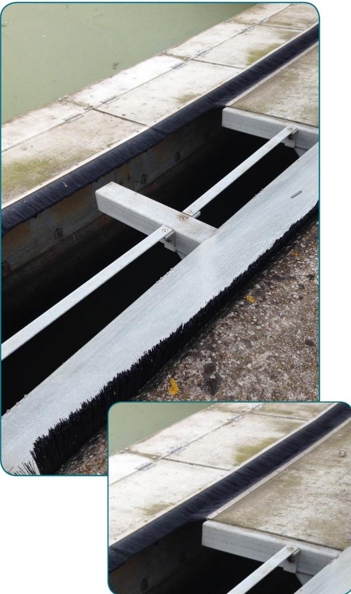
Figure 4: Covering on channel from inlet works to primary tanks
