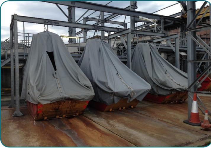
Figure 3: Brush covering on primary tank weirs
