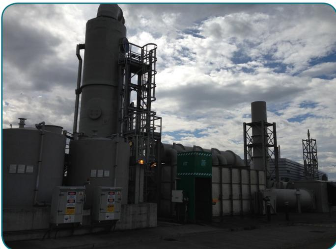
Figure 6: Activated carbon scrubber for air extracted from thermal hydrolysis sludge plant
