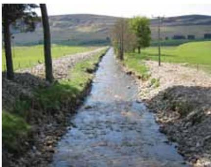
**The artificially straightened reach of the Rottal Burn in Angus, prior to re-meandering** (© Centre for River Ecosystem Science).
