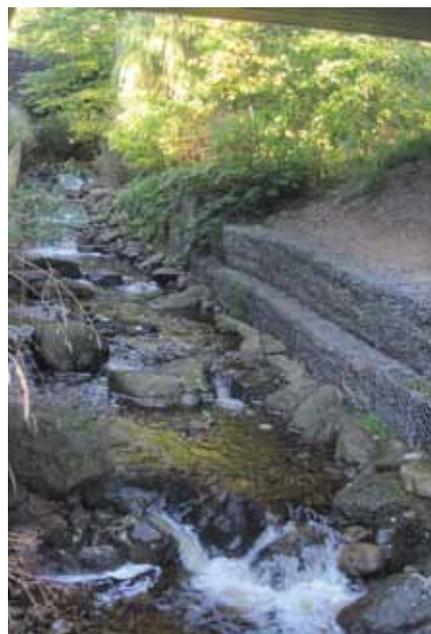
A reach of the Inchewan Burn, Perthshire, before and after replacement of the artificial bed with a more natural boulder and cobble substrate that restored fish passage to the upper catchment (© Centre for River Ecosystem Science).
