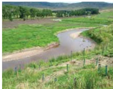
**The Rottal Burn in 2012 after re-meandering using the old course of the burn as a template** (© Esk Rivers and Fisheries Trust).
