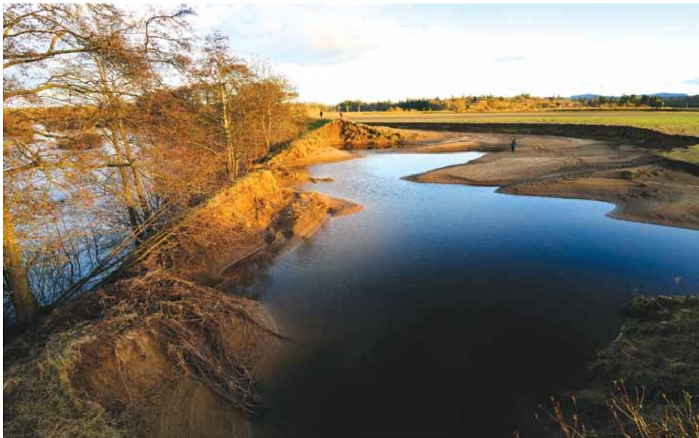
A breached flood embankment and scour hole caused by a large flood on the River Tay, Perthshire (© SNH).
