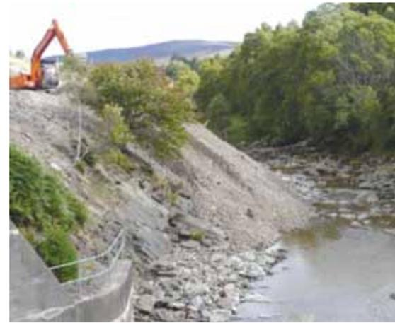
**Gravel replenishment on the regulated River Garry, Perthshire.** Gravel trapped behind a weir has been excavated and re-deposited below the weir to restore sediment supply to reaches downstream (© Chris Gibbins, Northern Rivers Institute).
