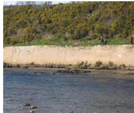
A previously eroding terrace bluff on the outside of a meander bend, stabilised by a concrete revetment to protect a nearby road (© The James Hutton Institute).
