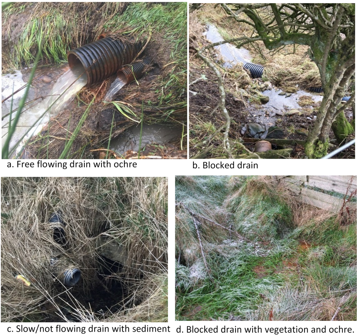
Figure 15 – Visual assessment of agricultural drains in ditches.
