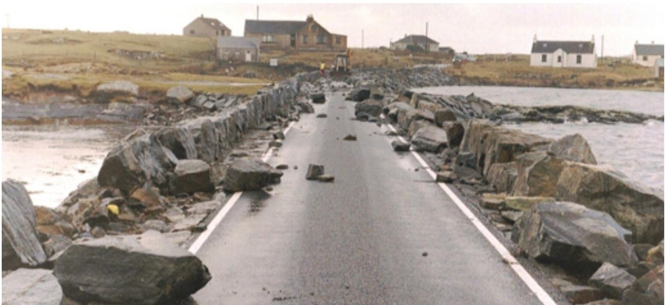
Figure 14: The storm of Jan. 11<sup>th</sup> 2005 in the Outer Hebrides presented major problems of how coastal communities adapt in response to extremes of climate change. Causeways that had been constructed to create an integrated transport network proved vulnerable to the effects of climate change.
