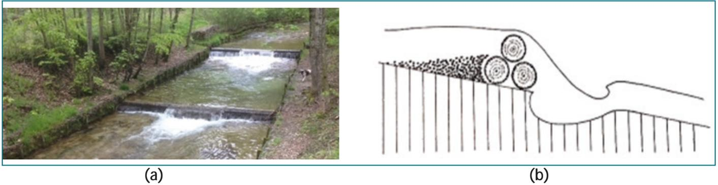
Figure 2.9: (a) grade control placement © C. Adams (b) cross-sectional view.
