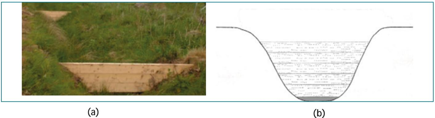
Figure 2.10: Ditch barrier placements (a) Belford project © Quinn et al., 2009 and (b) cross-section view.
