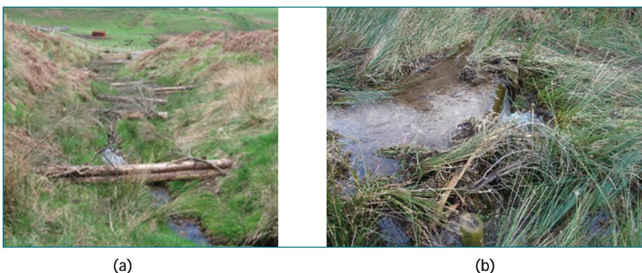
**Figure 6.2:** (a) Simple timber with low vertical height © S. Addy and (b) build up of sediment behind timbers creating a 'stepped' stream profile, similar to the effect created by grade-control placements © S. Addy.
