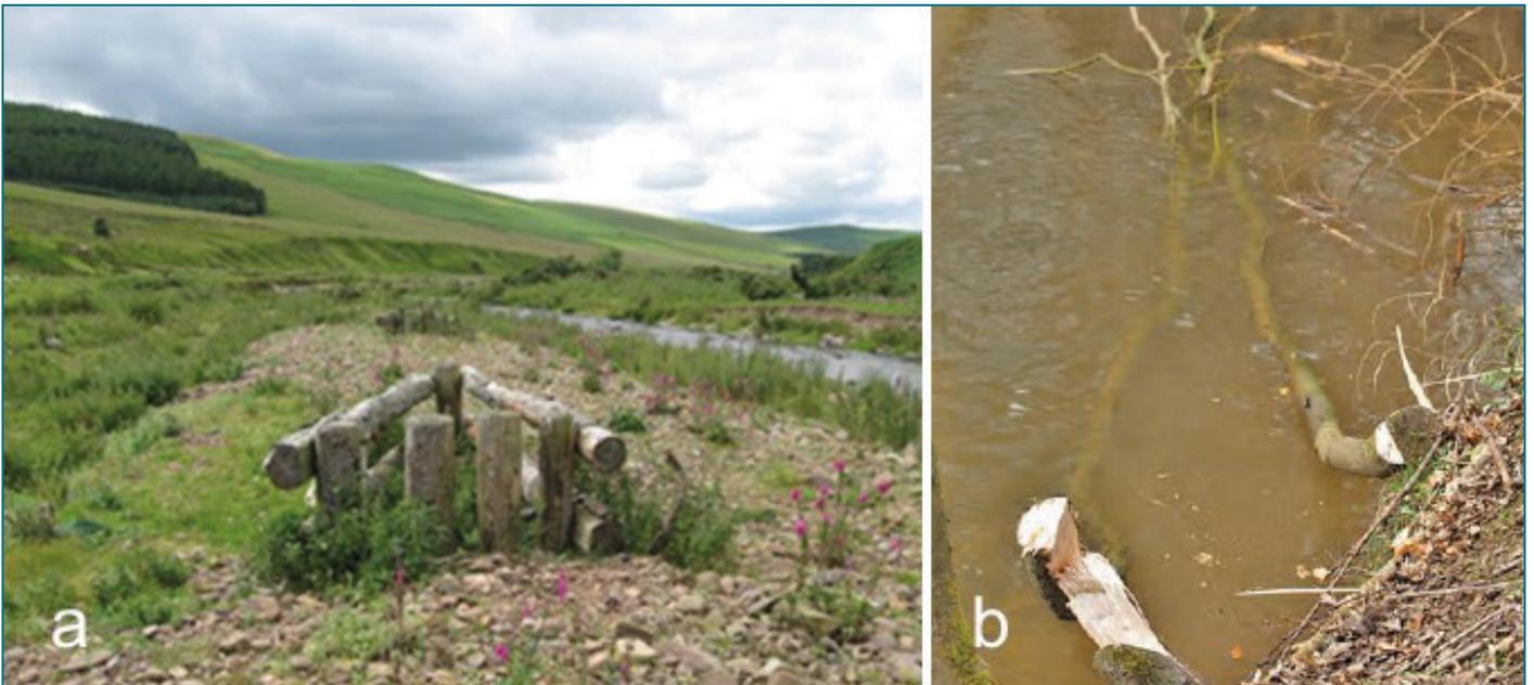
Figure 2.5: Examples of Category C placements (a) sidebar woody placements © S. Addy and (b) hinging trees © WTT, wildtrout.org.
