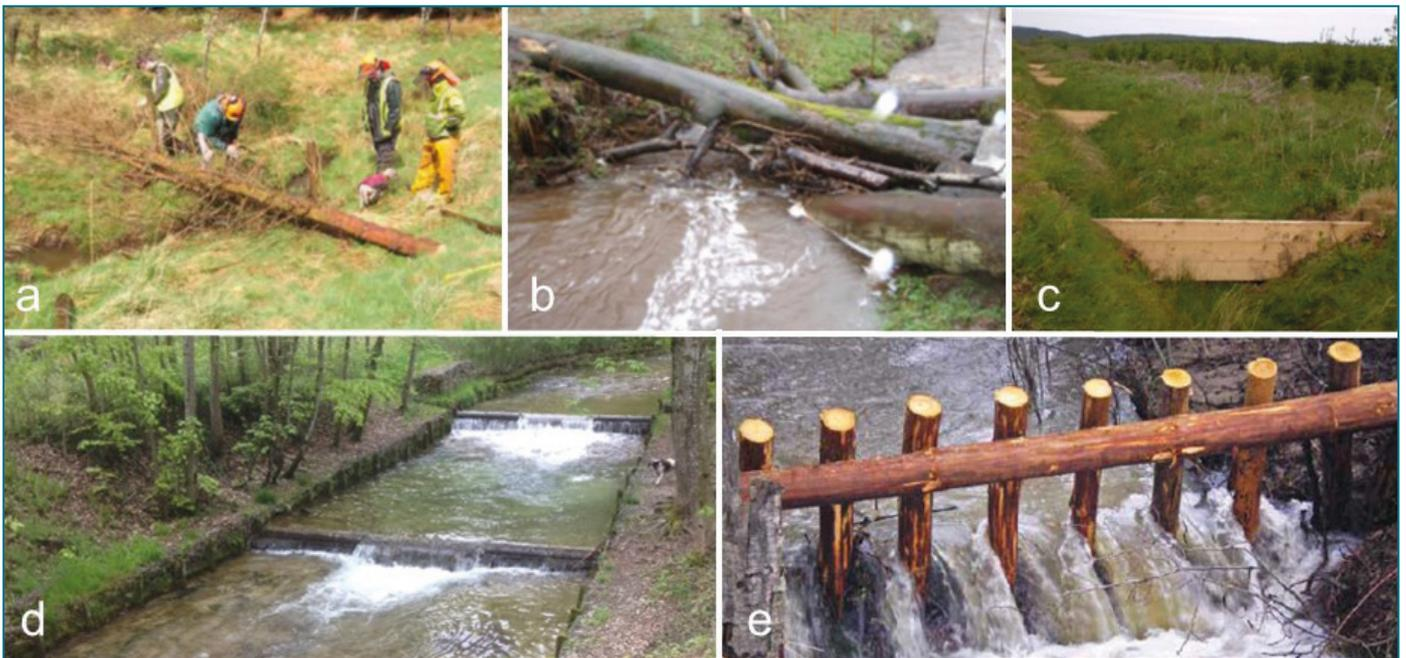
**Figure 2.4:** Examples of Category B placements arranged (a) complex single timbers © Tweed Forum, (b) man-made log-jams © Quinn et al., 2013, (c) ditch barrier placement © Quinn et al., 2013, (d) grade-control placement © C. Adams and (e) watergate placement © Kravčík, et al., 2012.
