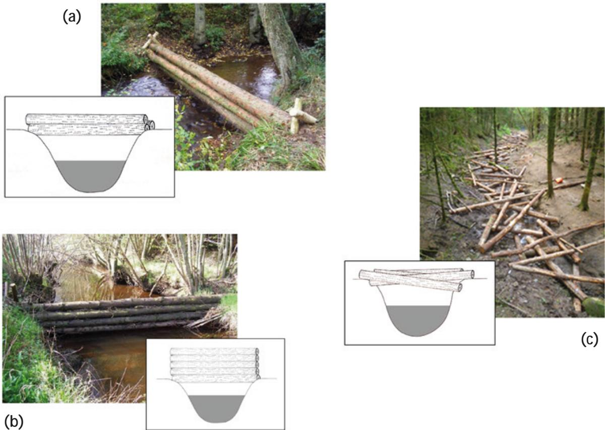
Figure 2.6: Examples of different types of Category A type placements. (a) simple timber with low vertical height © Nisbett et al., 2015 and schematic inset; (b) simple timber with high vertical stack height © Nisbett et al., 2015 and schematic inset; (c) lattice type placement © E. Starkey and schematic inset.
