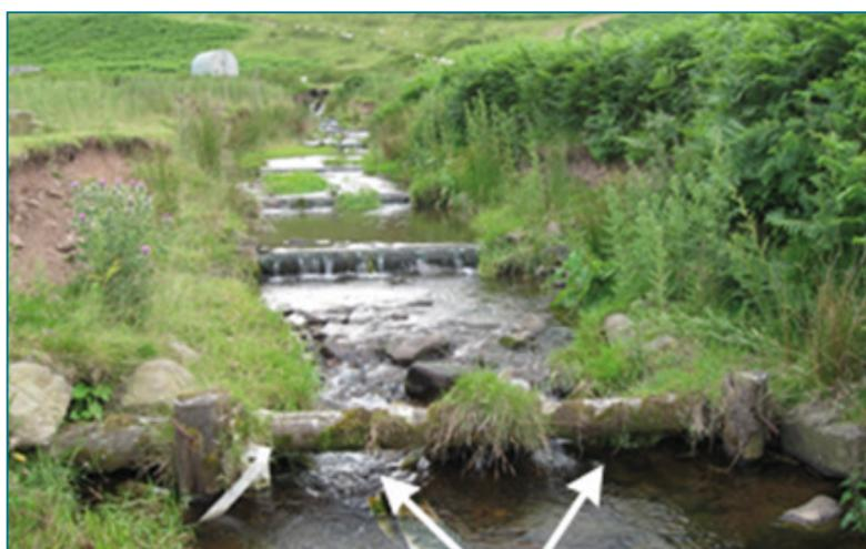
Figure 6.7: Under-scouring of grade-control placement (white arrows) © S. Addy.
