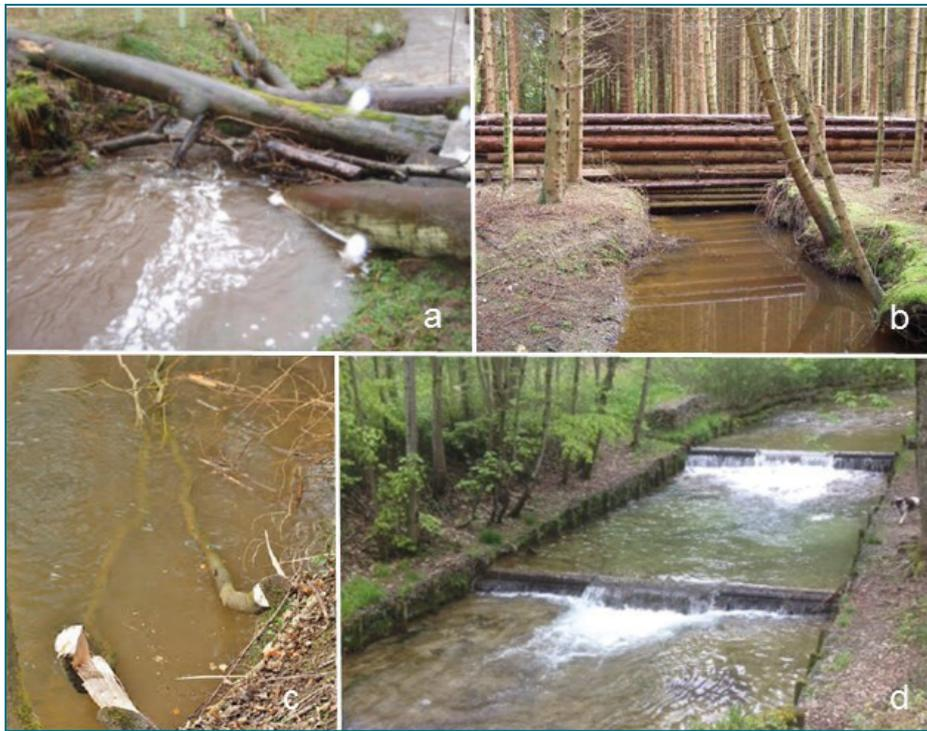
**Figure 2.1:** Array of structural woody placement types currently in use across the UK; (a) man-made log jam © Quinn et al., 2013; (b) timber bund © Nisbett et al., 2015; (c) hinged trees © WTT, wildtrout.org; (d) grade control placement © C. Adams
